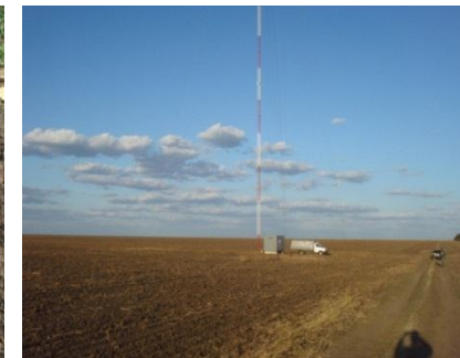
Met mast after installation
